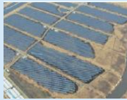
Solar power generation
