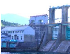
Hydropower generation plants
