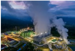
Geothermal power generation plants
