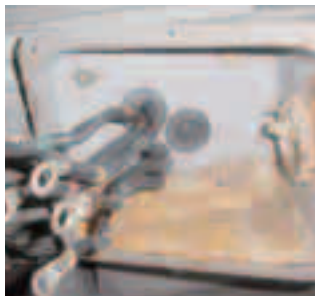
端子箱への水浸入 Water in the terminal housing
